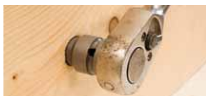
6. Release insertion sleeve with ratchet.
